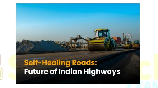
This technology will enable a road to 'repair' itself using a new type of asphalt. This material will be infused with steel fibre and bitumen. If a gap emerges on the road, the bitumen will spread to cover it and along with steel threads, fill the potholes.
