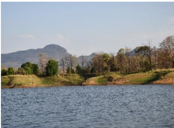
Back water of Tawa Reservoir
